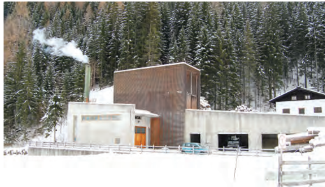
Heating plant in Sankt Nikolaus, Ultental, in Südtirol
